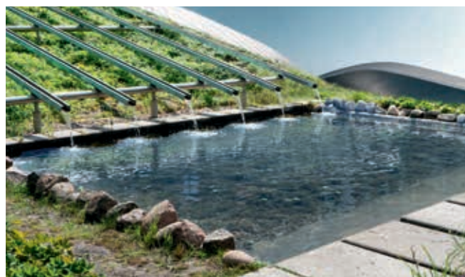
Fig. 23: Green and walkable roof terrace with pond irrigation system on an inverted roof with full gravel drainage layer.
