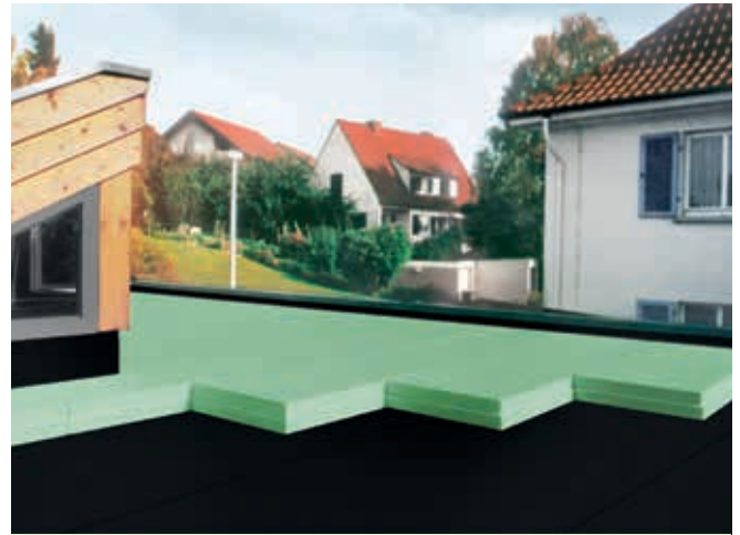
Fig. 25: Installation of Styrodur® boards under an extensive green roof.
