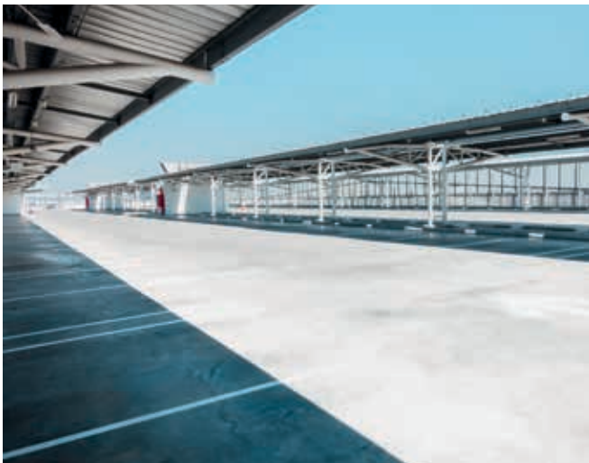
Fig. 49: Parking roof with in-situ concrete driving surface.
