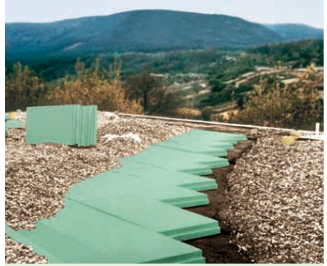
Fig. 16: Renovated inverted roof as a plus roof.
