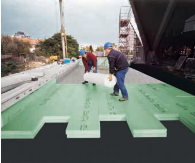
Fig. 15: Installation of Styrodur® on top of the roof waterproofing.
