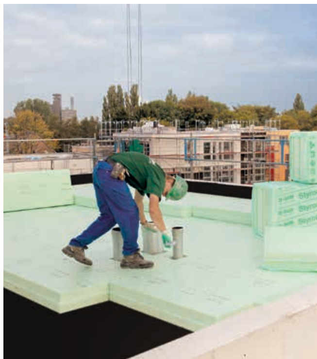
Fig. 3: Inverted roof insulation with Styrodur® for 250 housing units in Hamburg.
