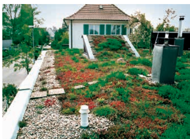
Fig. 35: Gravel strip along the roof edge and roof penetrations.
