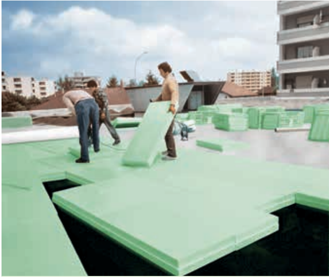
Fig. 12: Installation of Styrodur® for a duo roof.
