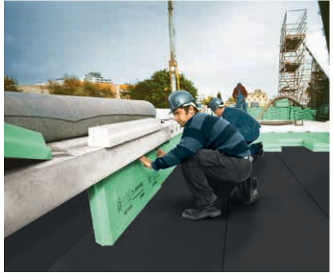
Fig. 13: Parapet insulation with Styrodur®.
