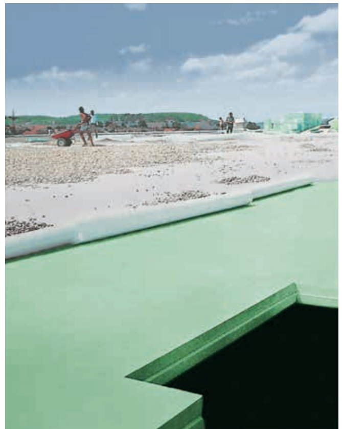
Fig. 9: Inverted roof with separation layer and gravel.
