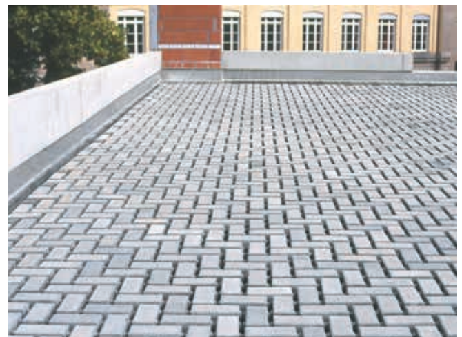
Fig. 47: Concrete pavement on Styrodur® boards.
