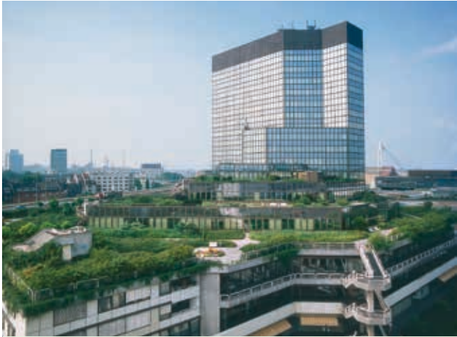
Fig. 27: Intensive green inverted roof.
